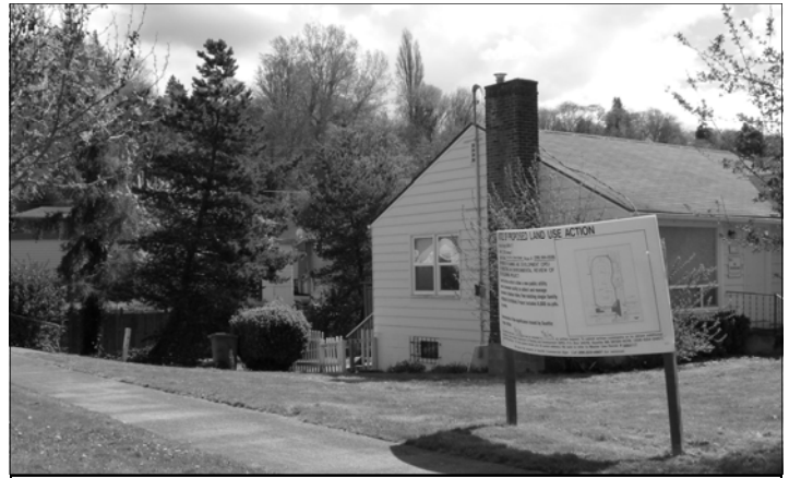
The flood site at 30th Ave E. and E. John St.
